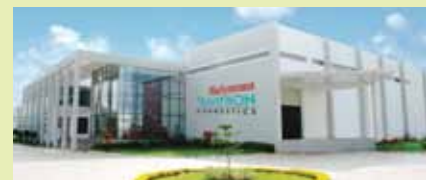
Biosystems Trivitron Diagnostic Solutions facility at Trivitron Medical Technology Park, Sriperumbudur, near Chennai.
